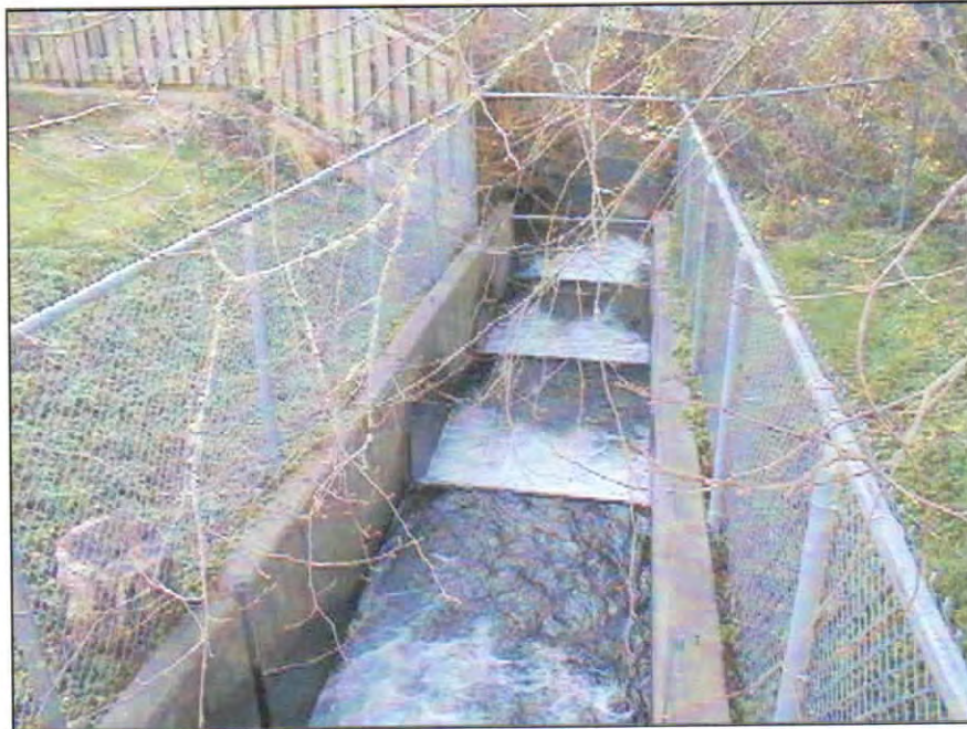
Figure 17 – Patterson Creek Fish Ladder at 9 th and Main
