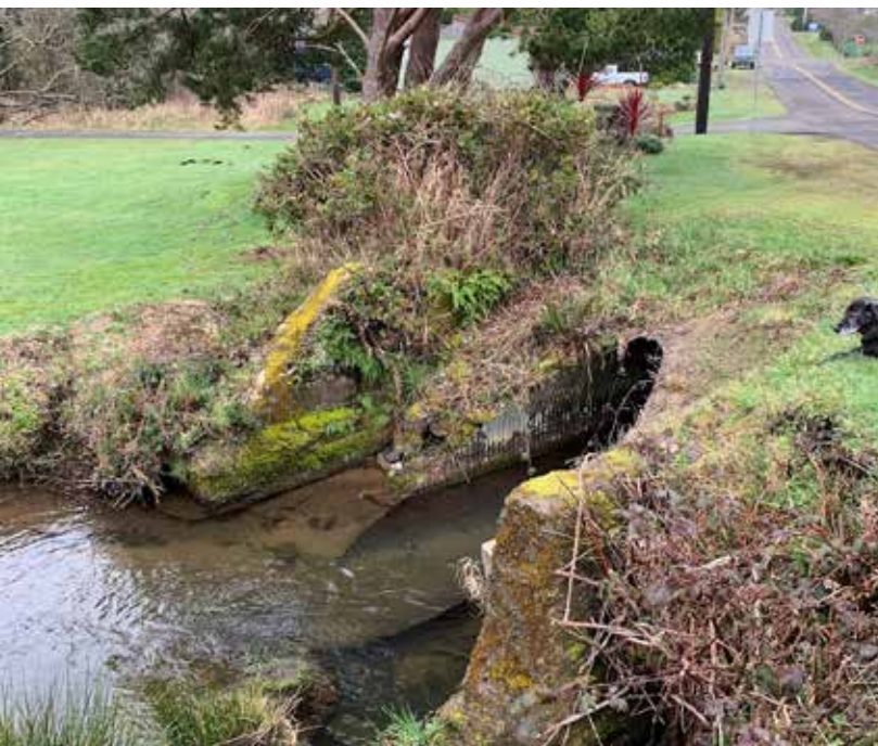
4TH STREET CULVERT
