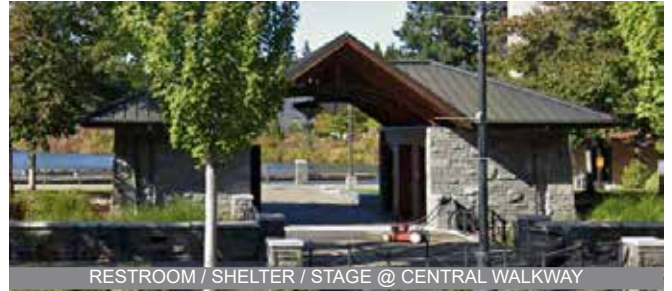
RESTROOM / SHELTER / STAGE @ CENTRAL WALKWAY
