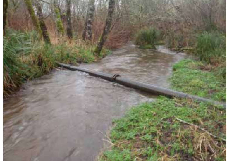
SEWER MAINLINE IN PATTERSON CREEK
