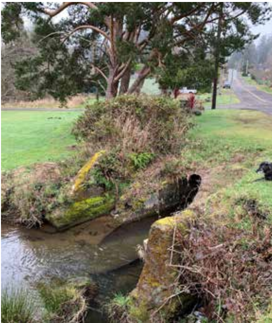
4TH STREET CULVERT
