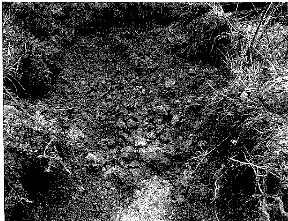
Photo 12 – View of the aggregate fill exposed along the edge of the main access road during test pit excavations.
