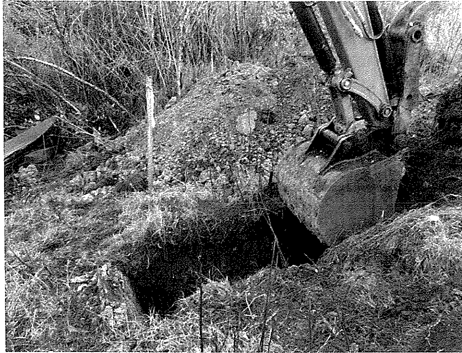
Photo 13 – View of Test Pit-3 during excavation.
