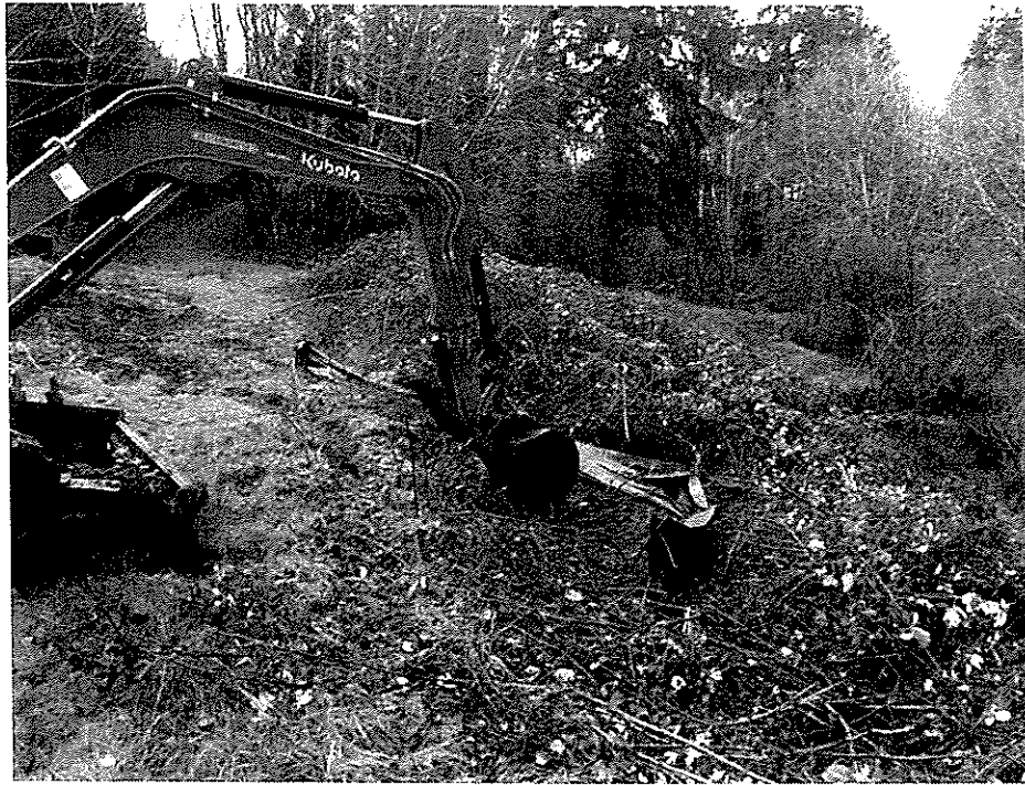
Photo 16 – View of Test Pit-7 during excavation.
