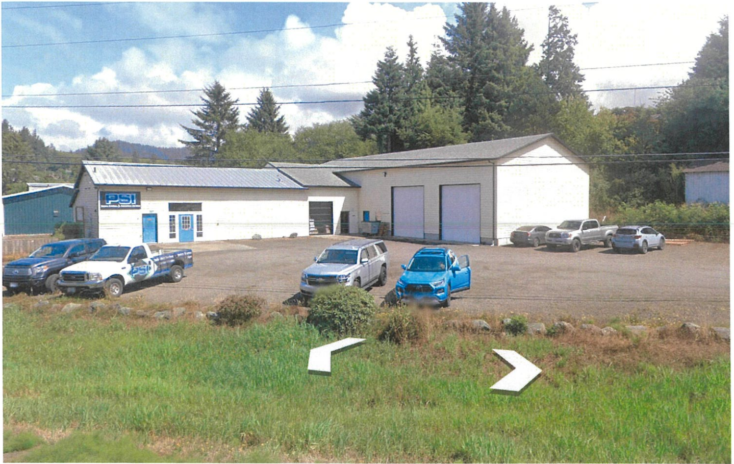
View of the Subject Property (looking north) from Highway 101
