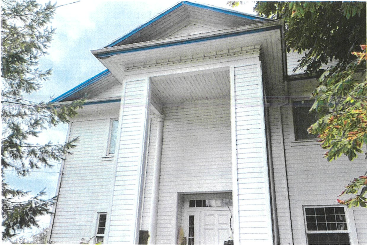
View from 5 th Street
