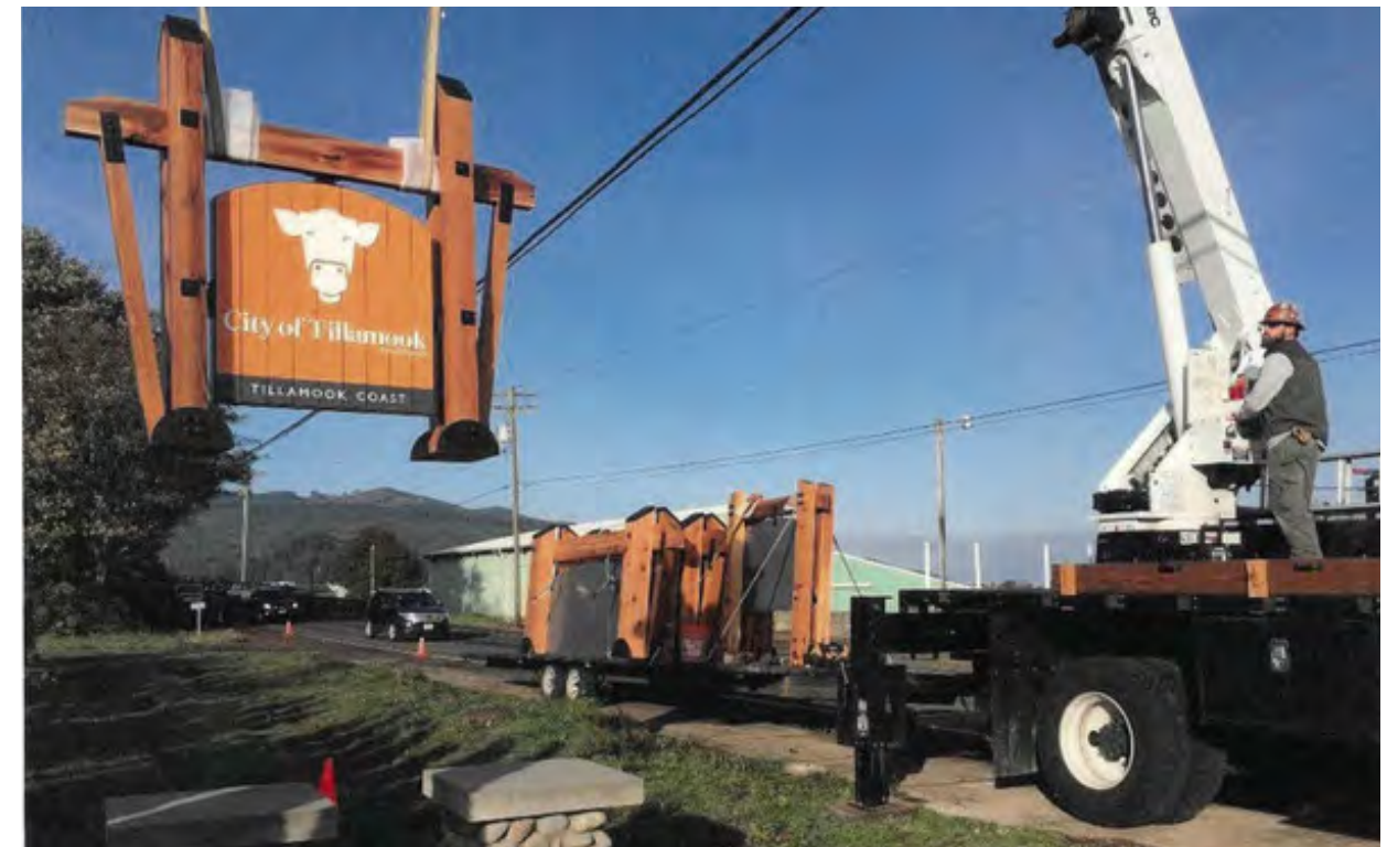
City of Tillamook Gateway sign installation.
