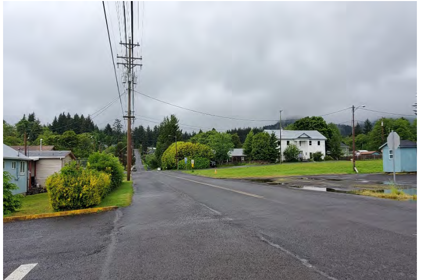
Current road conditions (Bay City)
