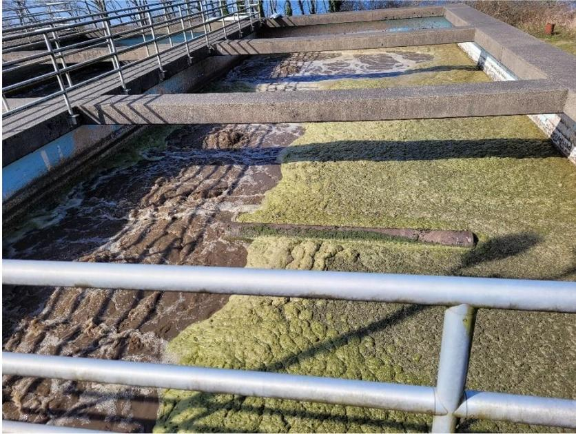
17: Aerobic Digester
