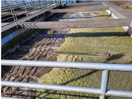
17: Aerobic Digester
