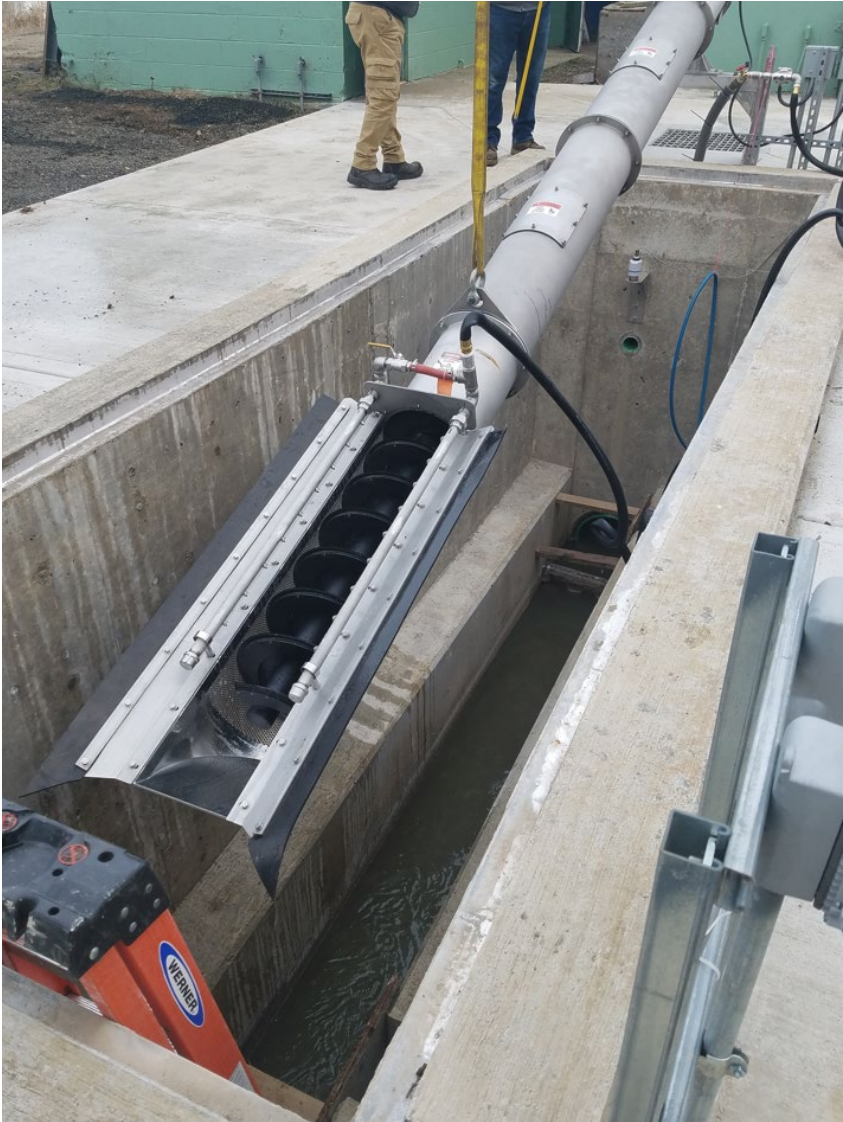
Screen being lowered into place
