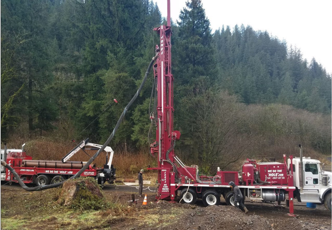
Well being drilled
