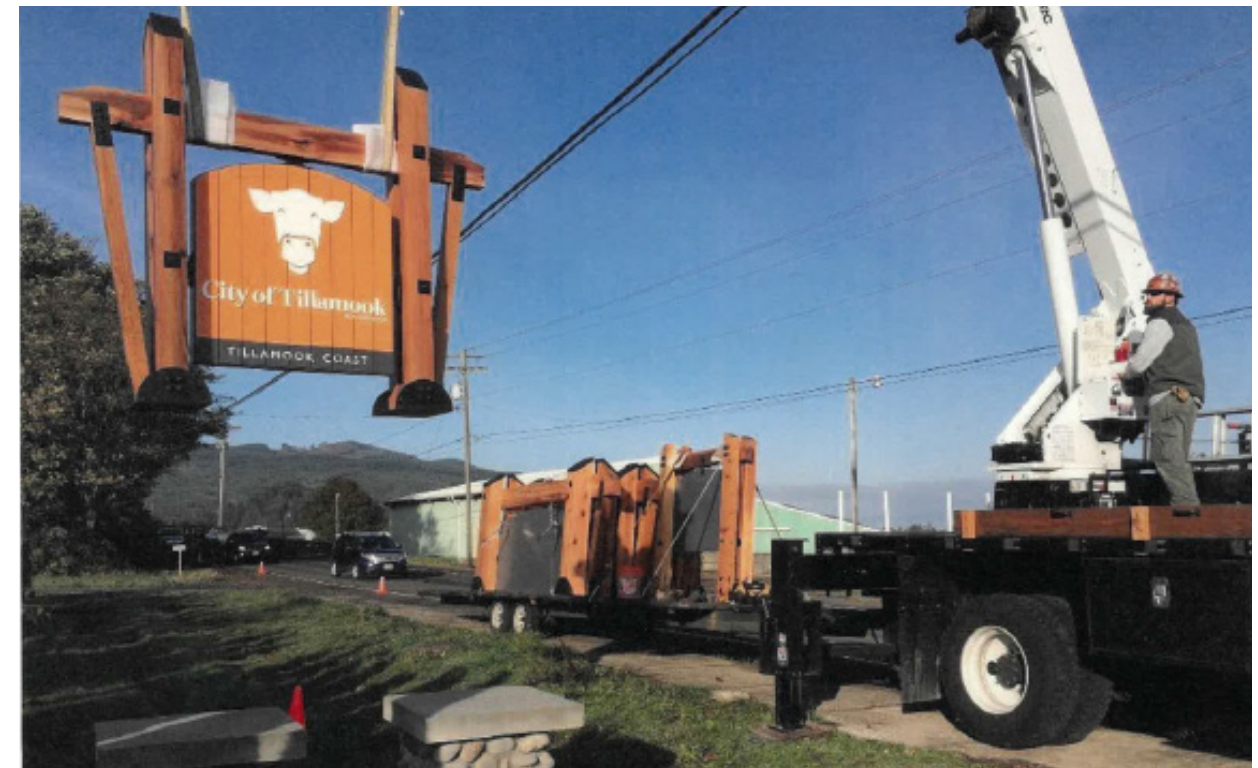
City of Tillamook Gateway sign installation.
