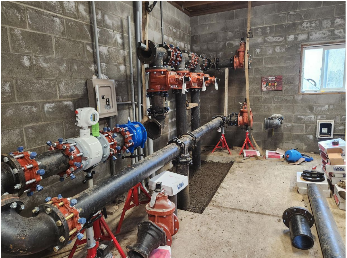
Well #3 piping tying the 3 wells together (not complete)
