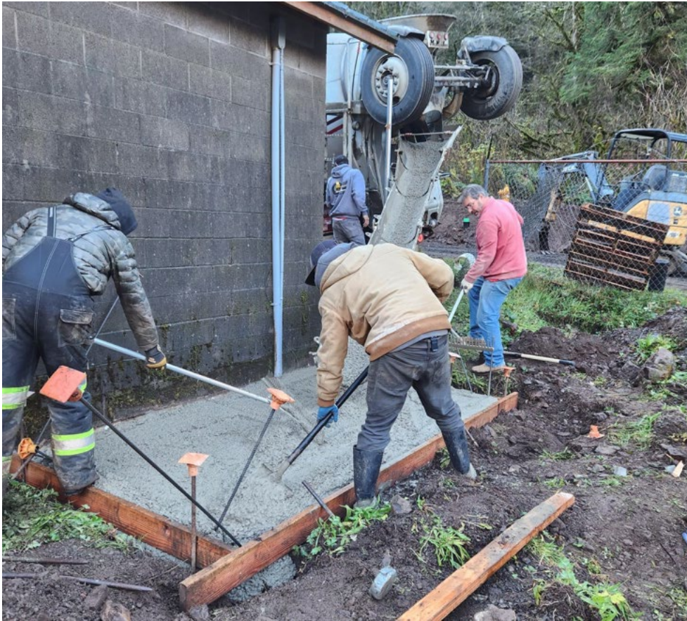
Floor for Chlorine Storage room at Wells
