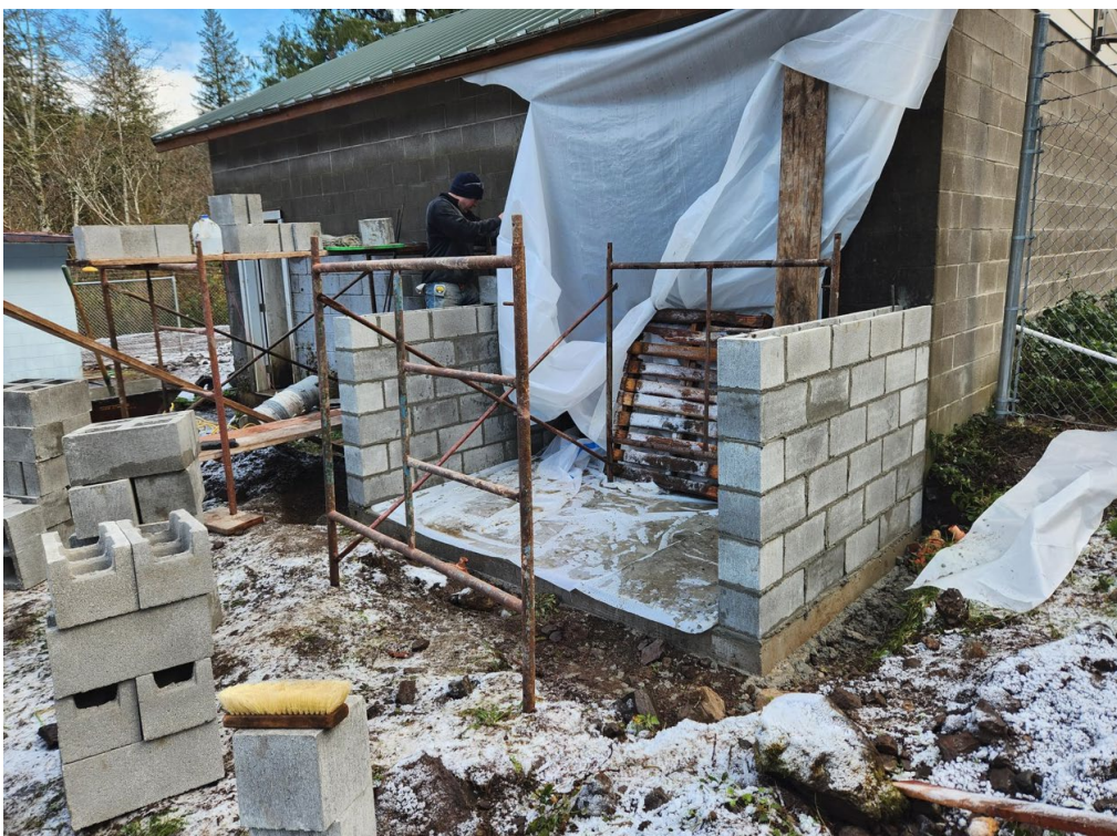
Walls for Chlorine Storage at Wells
