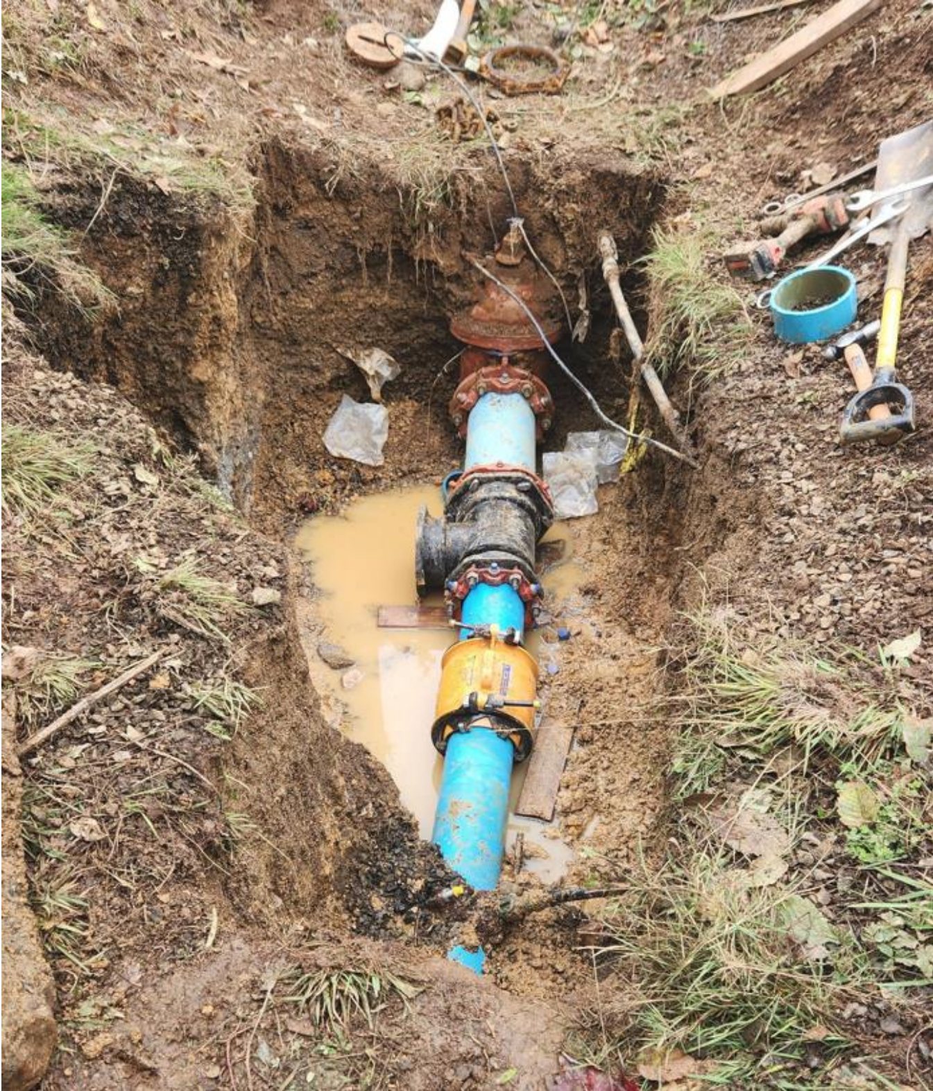
Partially installed Fire Hydrant on 7 th Street
