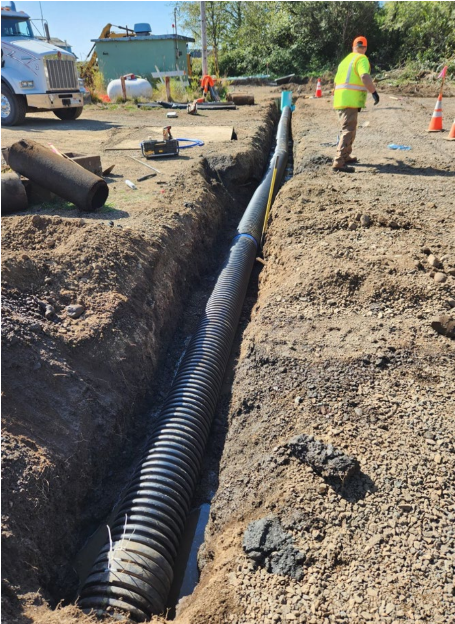
Storm pipe replacement
