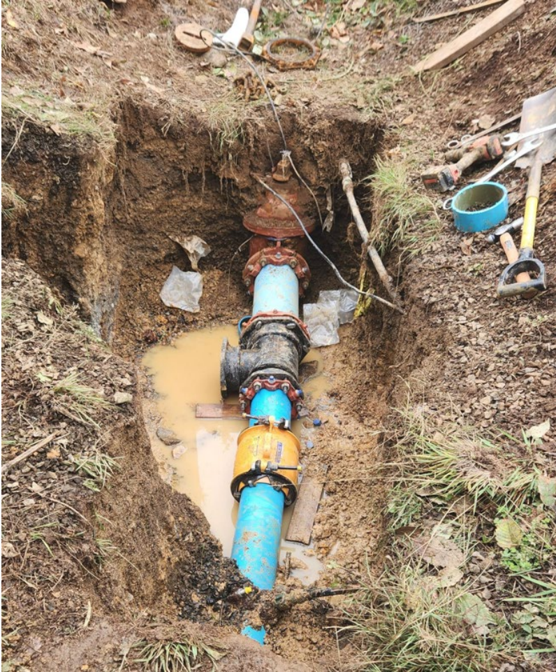
Hydrant being replaced
